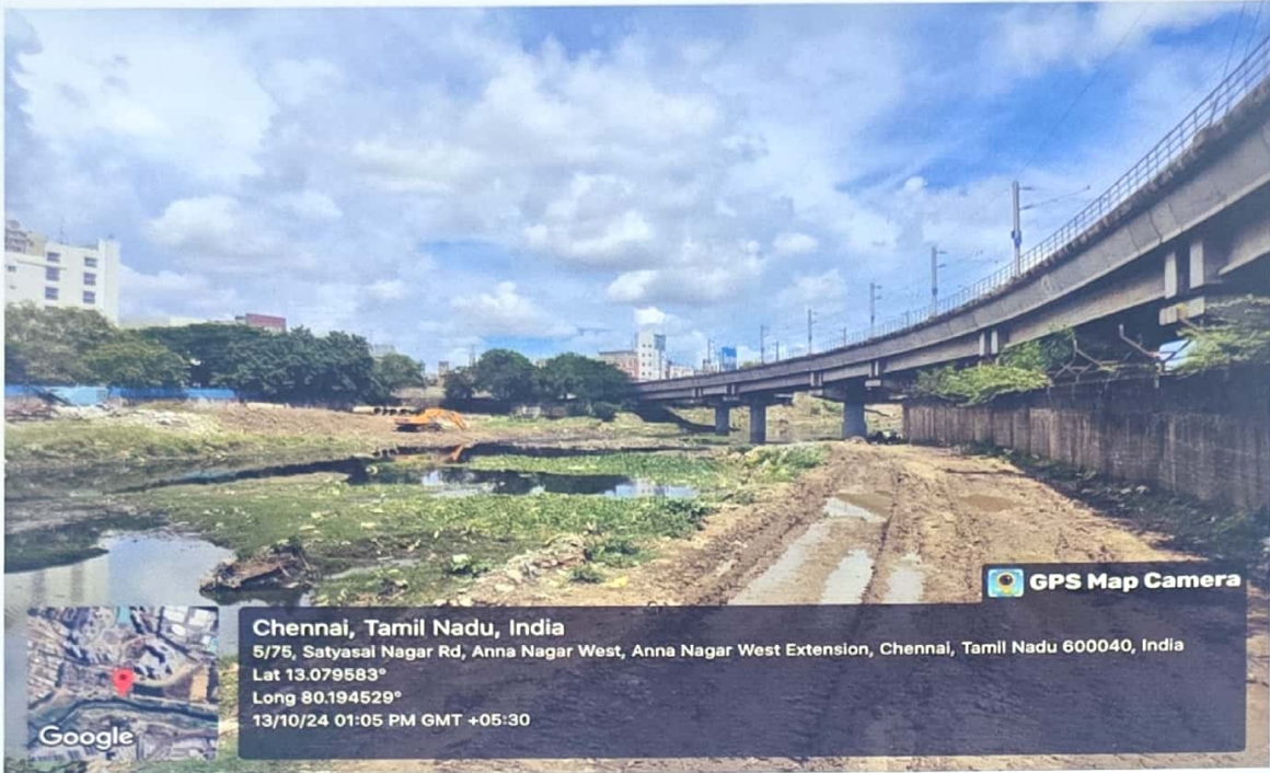
Inner Ring Road Up Stream (Near Sathya Sai Nagar)
